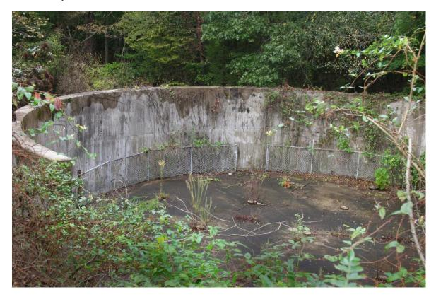
The semi-circular concrete block wall intended to contain the radiation being used on the cattle or other large animals while preventing inadvertent exposure in the direction of the lake that Joe Lenhard required be installed when the lake was created
